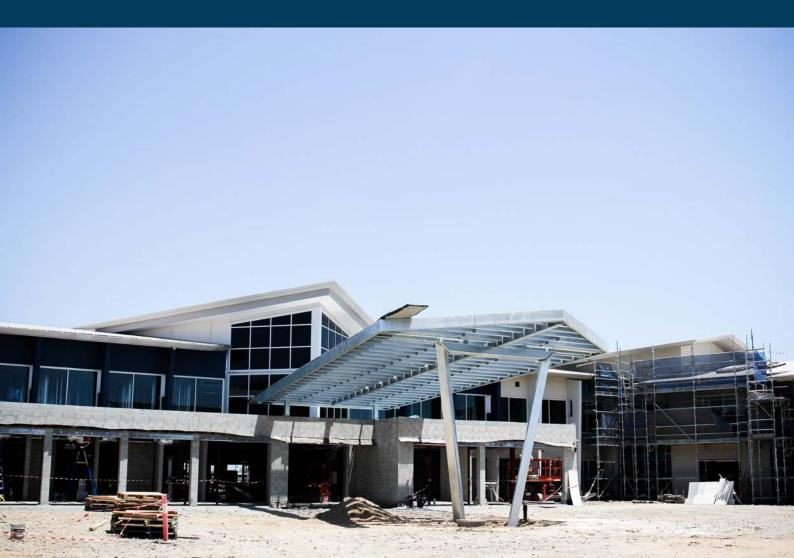
MSE delivered the structural steel package including the large Portico frame, located at the entrance. MSE took advantage of the well designed structure and built the roof frame on the ground which halved the construction time while also minimising working at heights, creating a safer workplace for all.
