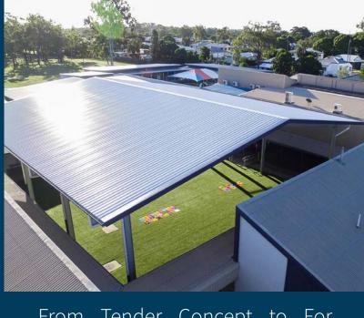
From Tender Concept to For Construction, our engineers were able to refine the steel design, by shaving a little over 2T of steel and approx. ~\$12k off our tender price, delivering a more economical build for the Client. Access was very tight and MSE designed the structure in a way that the Roof could be assembled in the carpark and lifted in one lift meaning Structural Steel Erection only took 3 days to complete allowing other trades to get in and complete their works on time.
